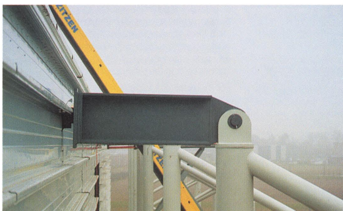
6. Connection details at roof level before the exterior cladding was put in place.
