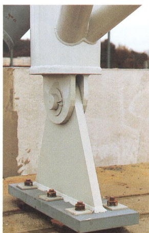
4. Spaceframe column connection to foundation.
